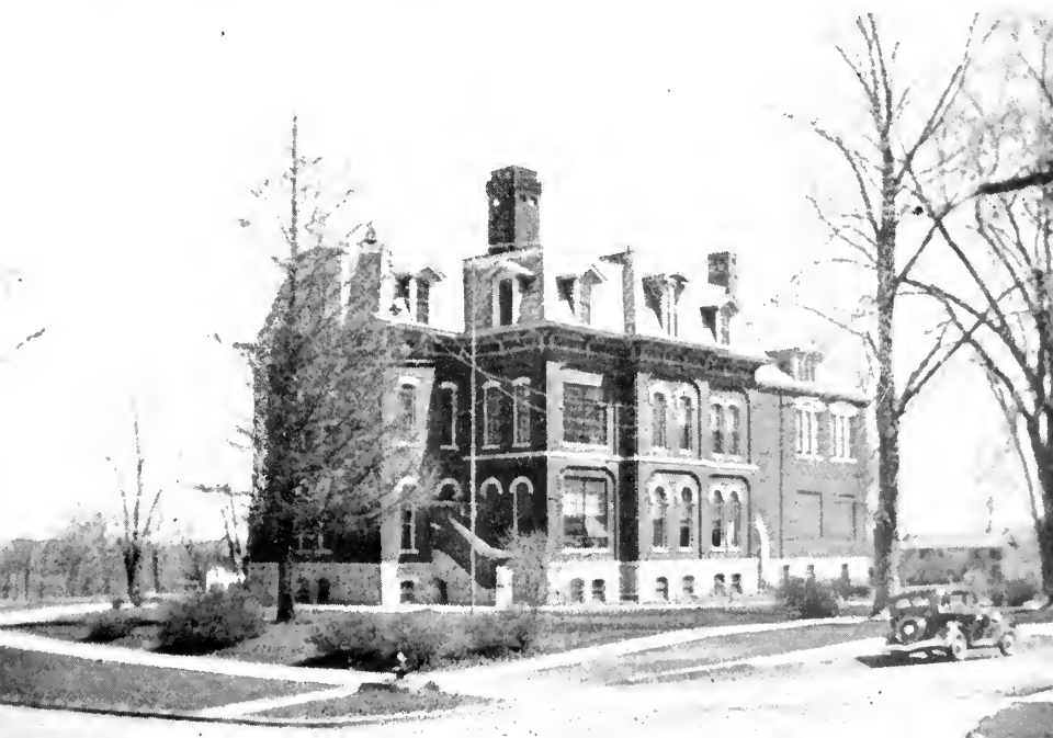
DELAVAN GRADE SCHOOL. A MODERN SCHOOL IN A BEAUTIFUL SETTING
